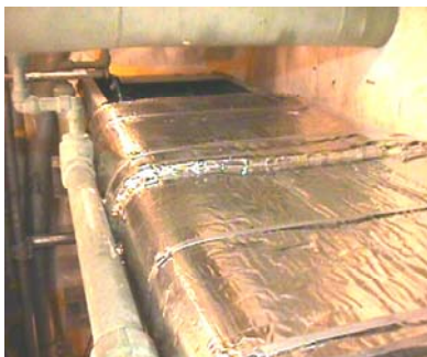
Shown above, the Interam™ installed as a one-hour fire barrier.
